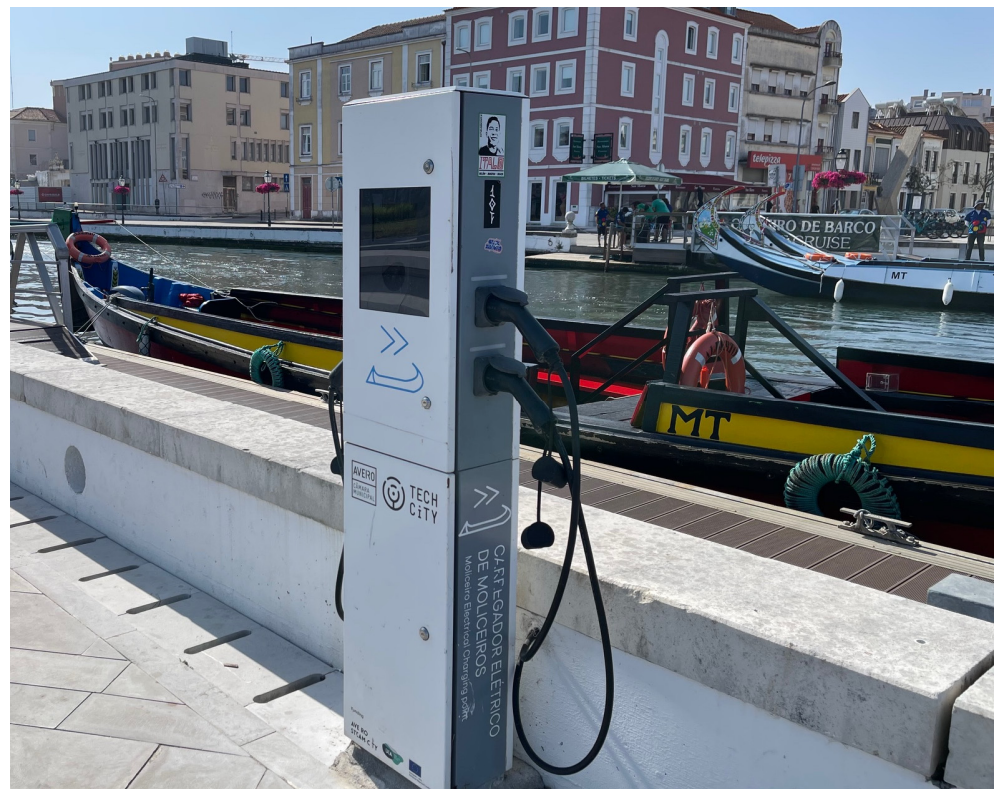
Figure 5. In-place electric charging station for ‘moliceiro’ boats (in context).
